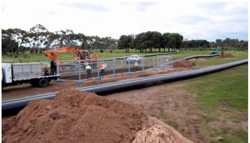
*Above: Four lengths of 240m long pipes of 650mm diameter were deposited in the south Parklands in early June. Installation work finished at the end of July and some remediation continued into August.*
