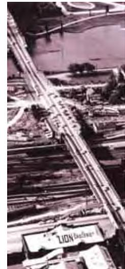
(Above) Prestressed concrete bridges replaced the Victoria Bridge across the river and the steel lattice bridge across the railyards; the original Lion factory is in the foreground – the eastern (right hand) section was demolished to make room for the new bridge
